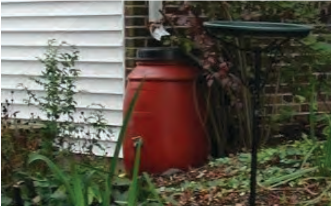
Rain barrels, such as this one at DWRC's Newark campus headquarters, can help control rooftop runoff
