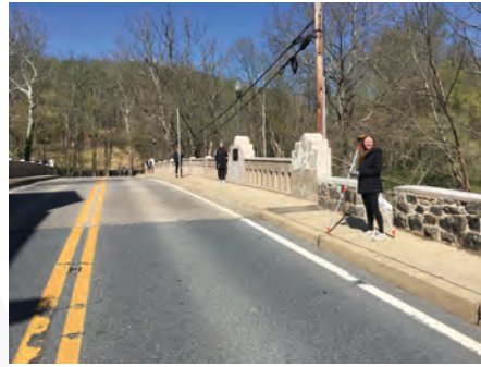
CIEG 467 667 Streampower Field Survey Rockland Rd. Bridge on the Brandywine (Apr 8, 2025)
