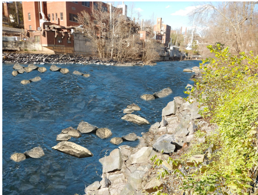
Dam 6 Removed and Channel Restored
