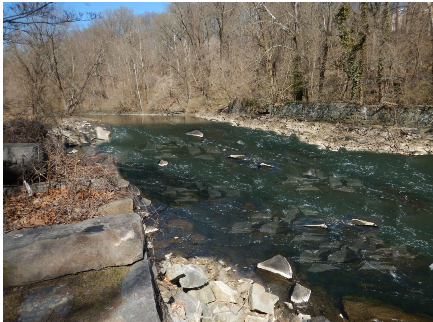
Dam 3 Removed and Channel Restored
