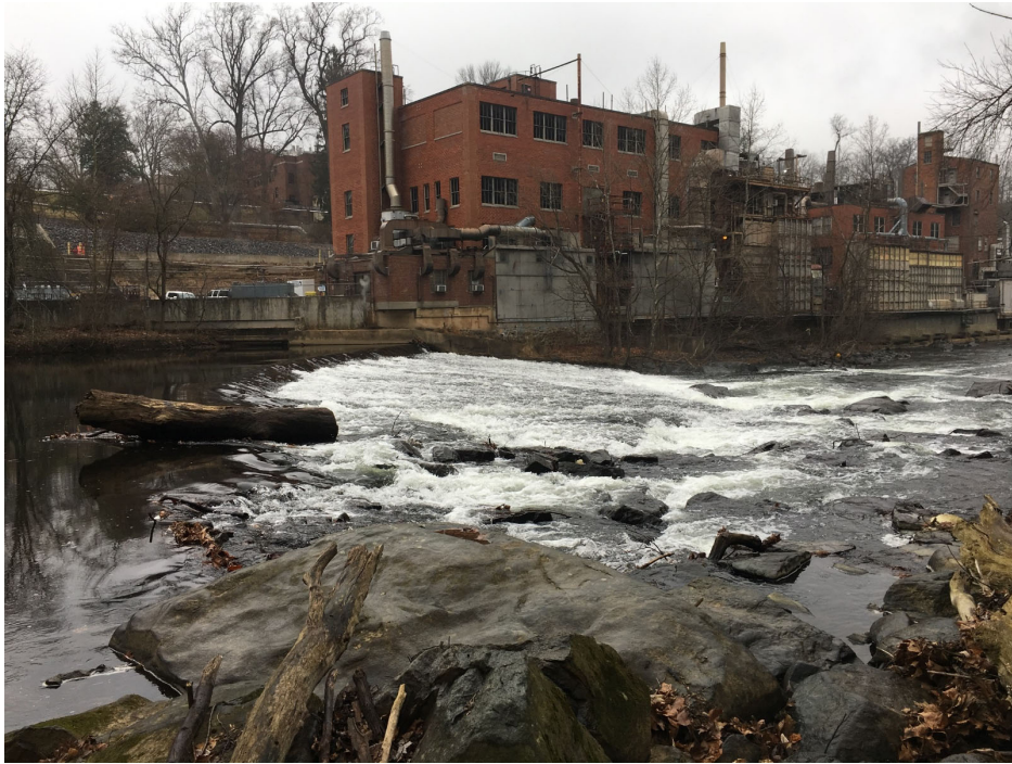
DuPont Dam 6, breached
