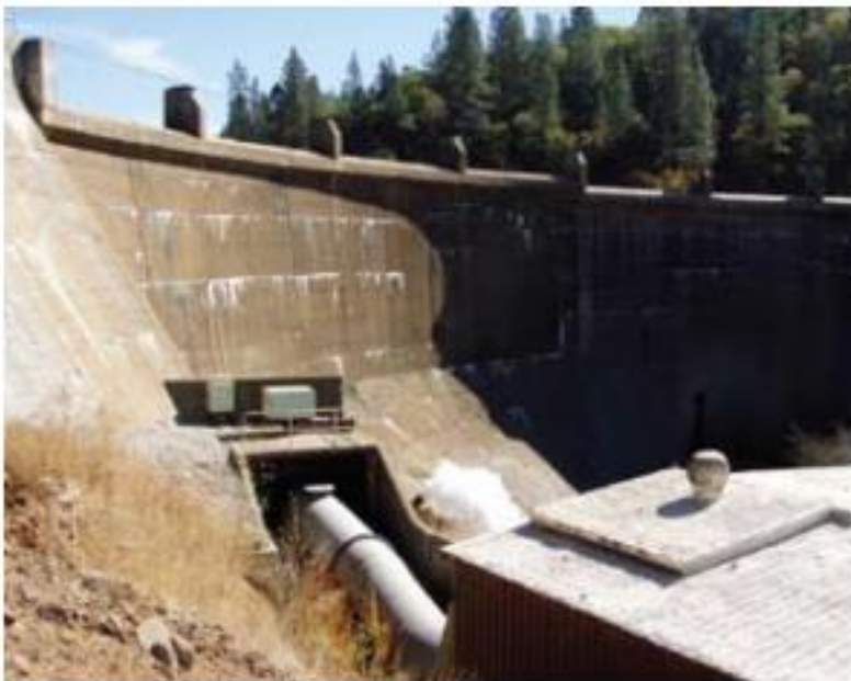
Figure 2: Combie Reservoir Dam
